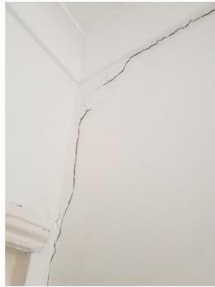
Image 01- Wall cracks due to ground instability
